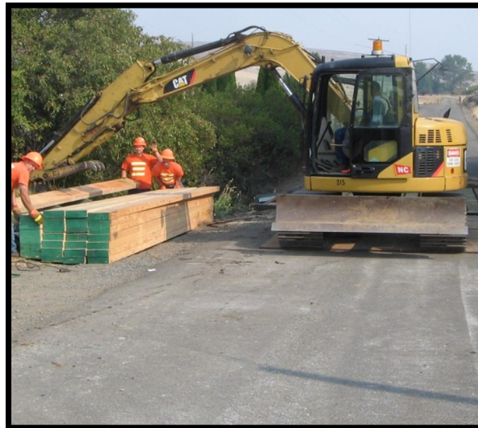
Crew at work on Glover Rd bridge
