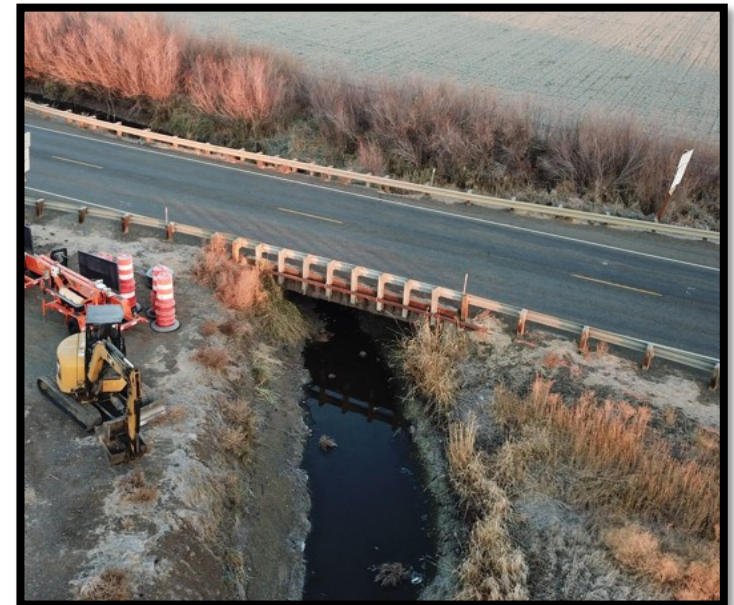
Vantage Hwy over Cascade Canal
