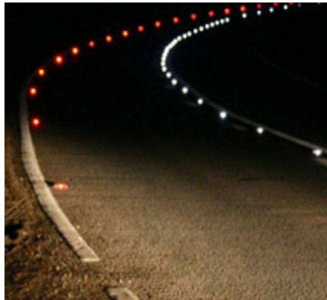
Embedded roadway lights
