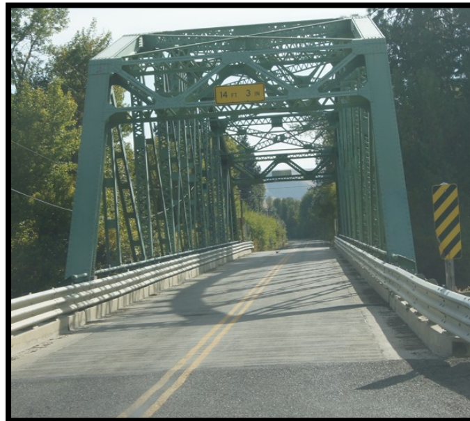
Thorp Hwy bridge over the Yakima River
