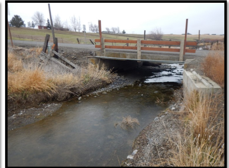
Bridge deck elevation looking south
