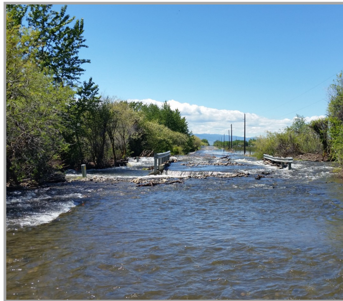
Flood event of 2017; overtopping bridge.
