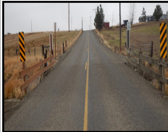
Hungry Junction Rd bridge deck looking east
