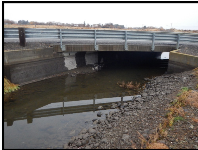
Reecer Creek Rd bridge deck looking east
