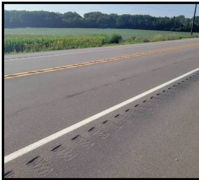
Installing rumble strips
