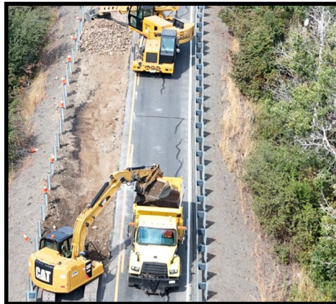
County forces repair of Teaway Road in 2025
