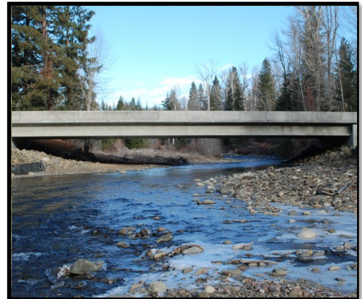
West Fork Teanaway bridge
