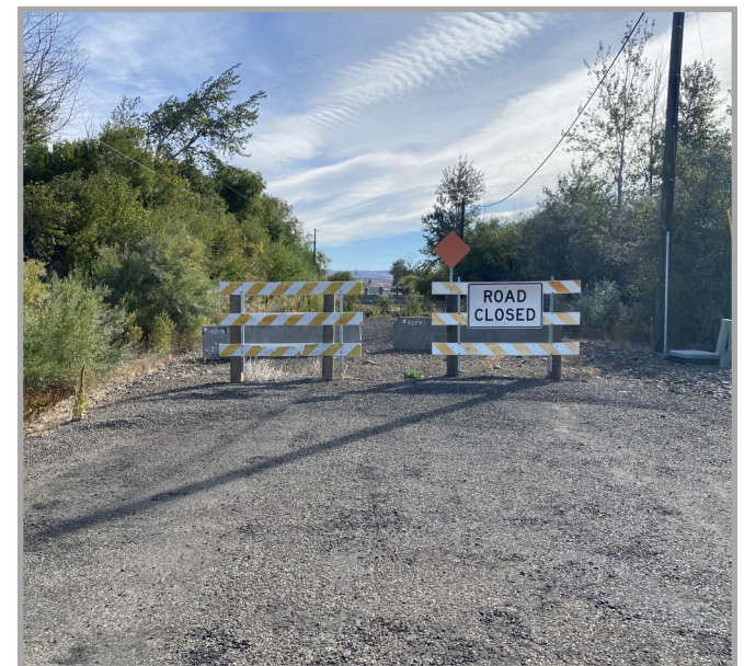
Bar 14 Rd with barricades after bridge removed.
